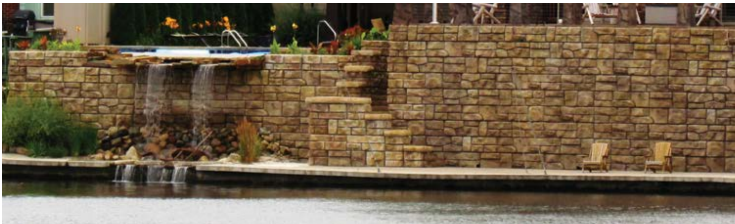
Figure 34 - Water feature part of Redi-Rock wall
