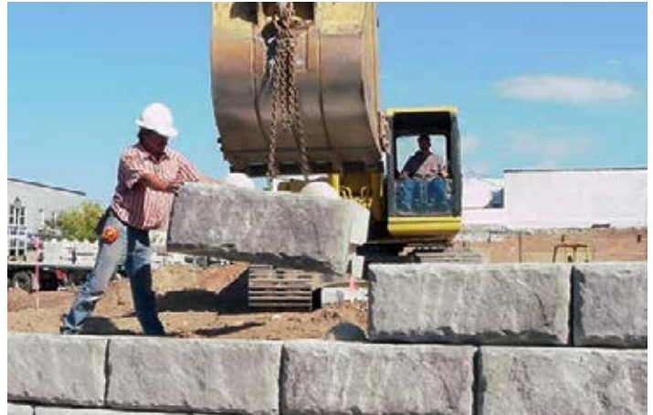
Figure 8 – Excavator Placing a Block
