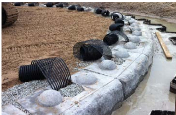
Figure 20 – Installed Drainage Aggregate
