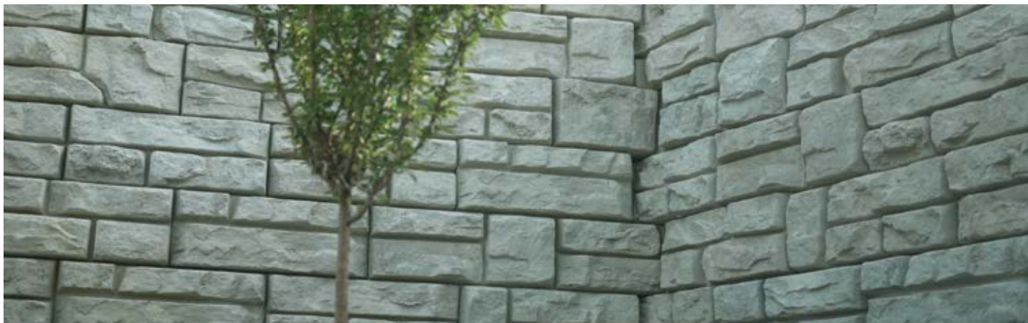
Figure 32 – Inside Corner of a Redi-Rock Wall
