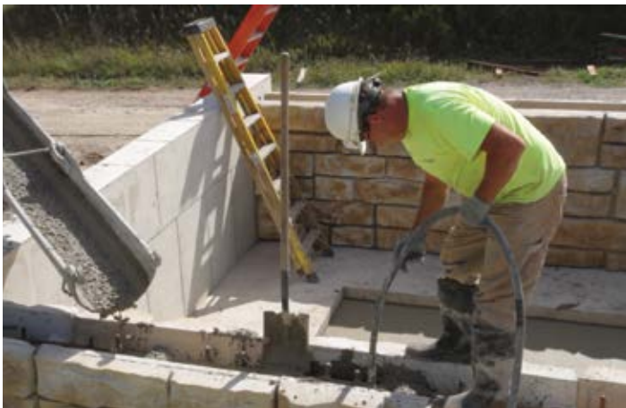
Figure 28 – Fill Hollow Core with Cast-In-Place Concrete
