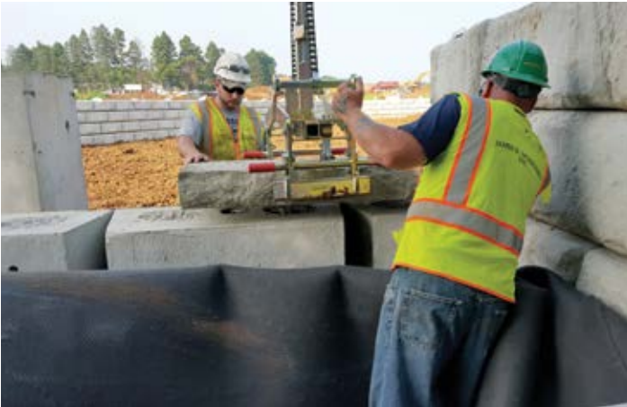
Figure 30 – Installing Cap on Retaining Block
