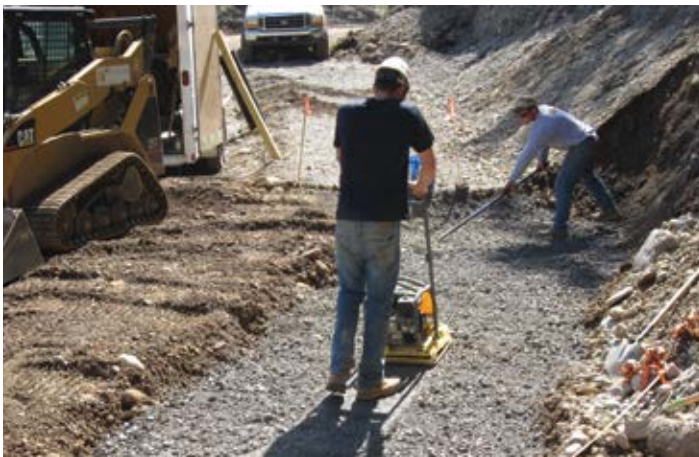
Figure 3 – Walk-Behind Plate Compactor on Subgrade Soils
