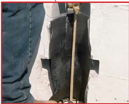
Figure 11 – Placing Non-Woven Geotextile Fabric
