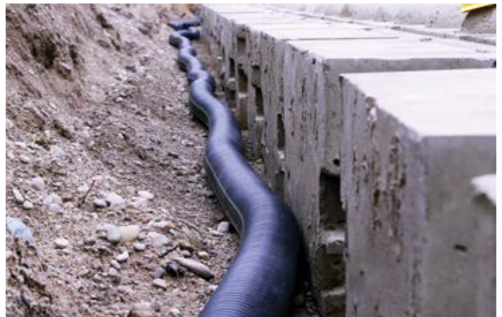
Figure 14 - Placing the Wall Drain
