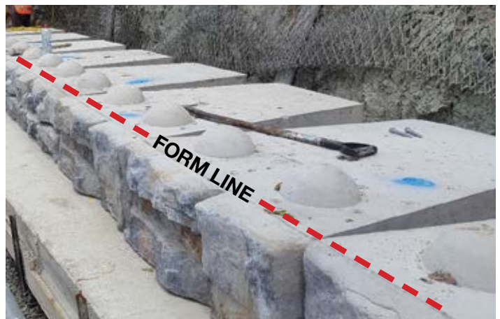
Figure 10 - Form Line Alignment
