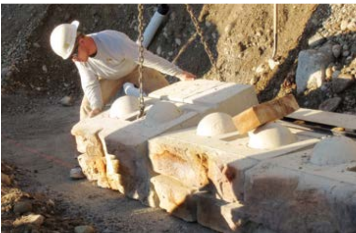
Figure 9 – Placement of Bottom Row of Blocks on the Leveling Pad
