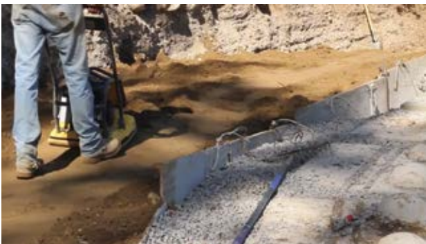
Figure 12 - Walk-Behind, Vibrating Plate Compactor
