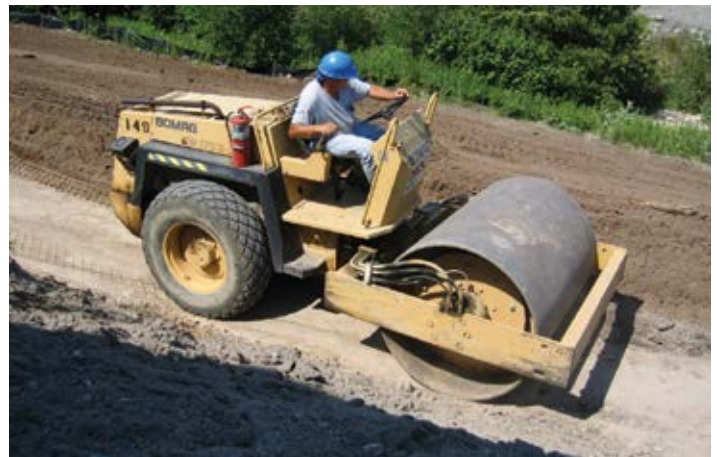
Figure 4 – Mechanical Compaction/Road Roller (Not Shown in Subgrade Application Here)
