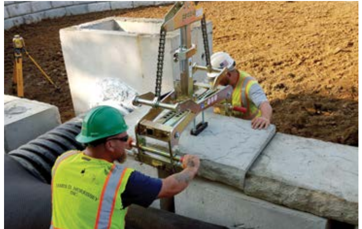
Figure 31 – Installing Cap Using Clamp
