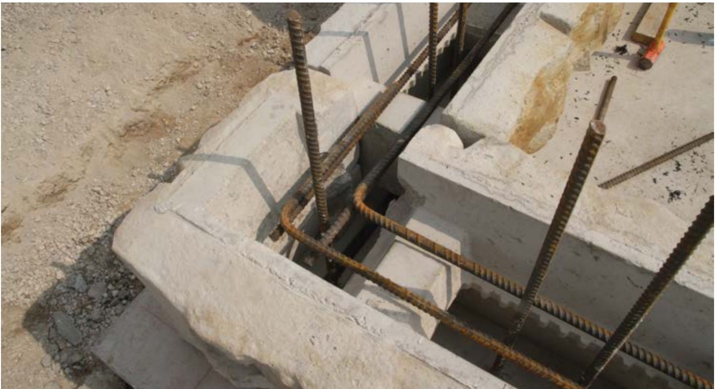
Figure 27 – Rebar in Grooves Ready for Concrete Fill
